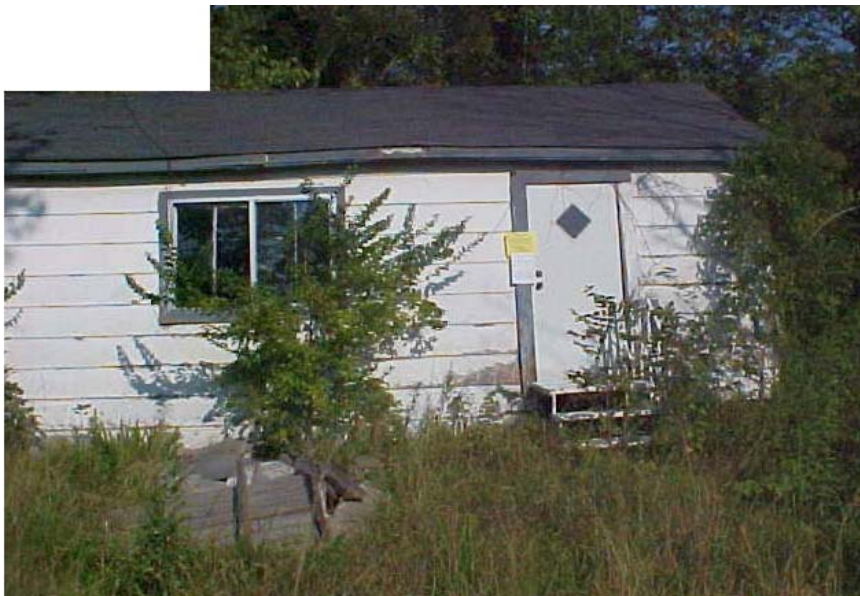
Front view of structure to be removed
