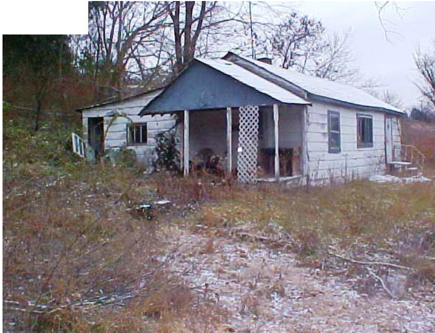
Side view of structure to be removed
