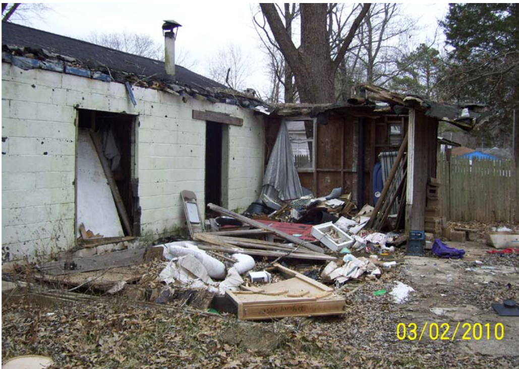
Back side of structure to be removed
