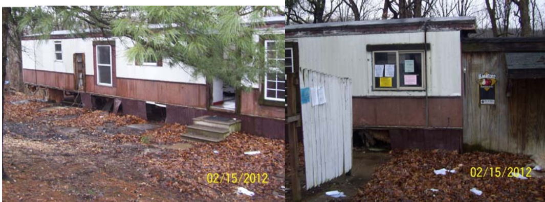
Mobile home to be removed
