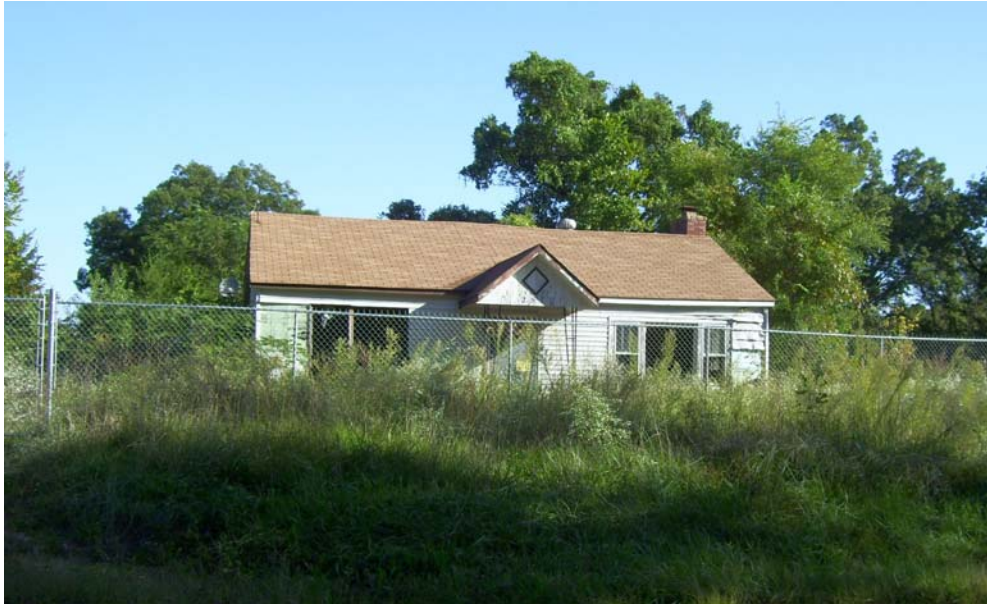
structure to be removed
