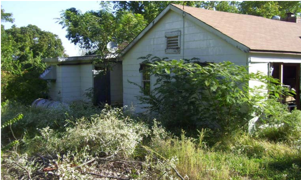
side view of structure to be removed
